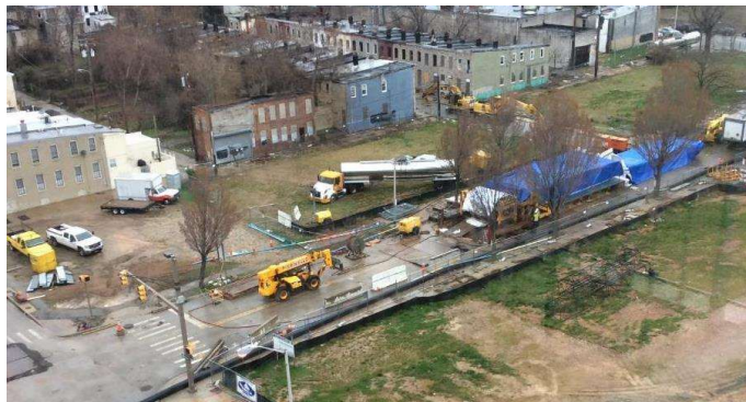
10' Diameter CIPP Wet Out Footprint – 3 to 4 traffic lanes
