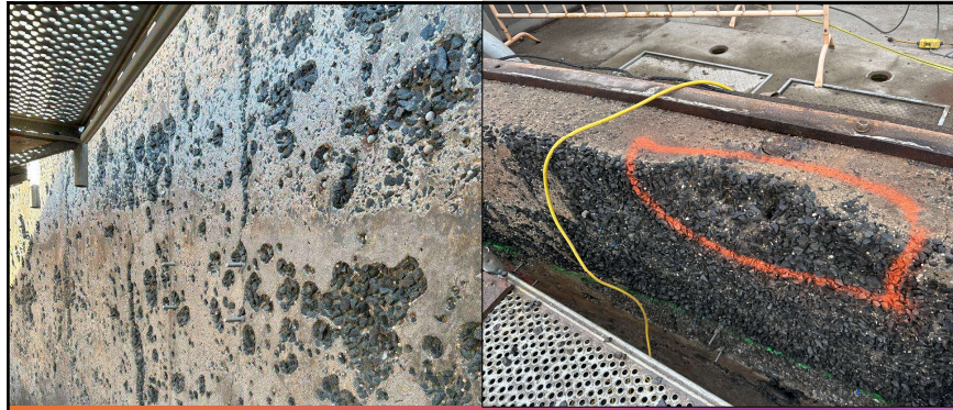
Decant Tank 3 – Larger Repair Pockets
