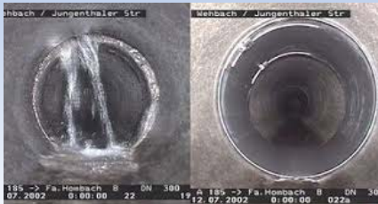
Stop Water prior to lining
