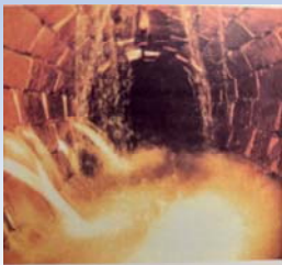
Infiltration Gusher- Maybe Grout or QL Prior to lining
