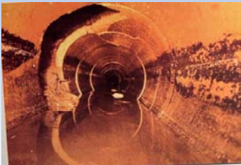
Hole in Pipe Visible Void – May need QL Sleeve prior to lining
